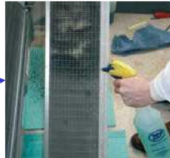
4. AC Clean Sanitizer is excellent for cleaning and sanitizing filters. The product can be sprayed on the filter or the filter can be dipped in the product.
