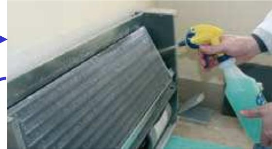
2. Spray the solution on the fin fan cooler surfaces starting from the top
