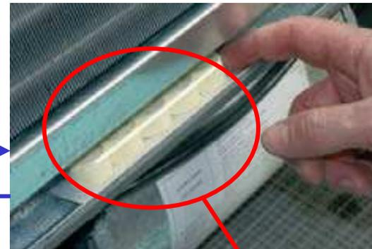
**4.** Insert the 5 tablets in the highest part of the condensate collector
