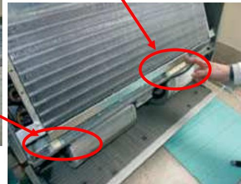
**6.** The tablets must be positioned at opposite sides of the drain pan.
