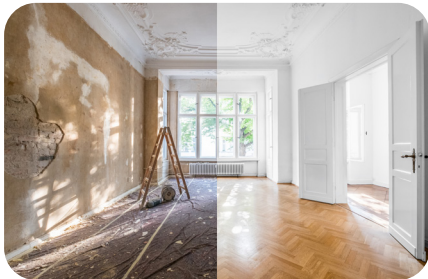
The upgrading of existing buildings
